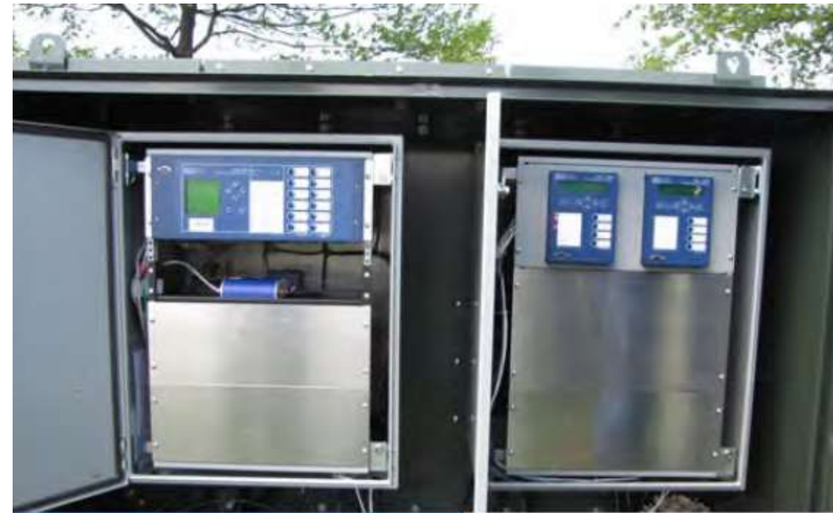
NEMA 4 OR 4X CONTROL ENCLOSURE (LOCATED THE SWITCH ENCLOSURE)
